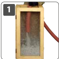
Dry injection with hose
