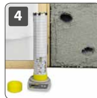
Testing the density of the filled test element with the NW100 density testing set.
