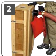
Dry injection with ventilated rotary nozzle
