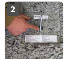
Testing the thickness of open blown insulation with the thickness gauge.
