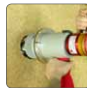
Injection of insulation
