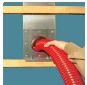
Insertion of the injection hose
